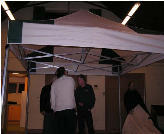
Roof panel fitted and the upper frame being expanded.
