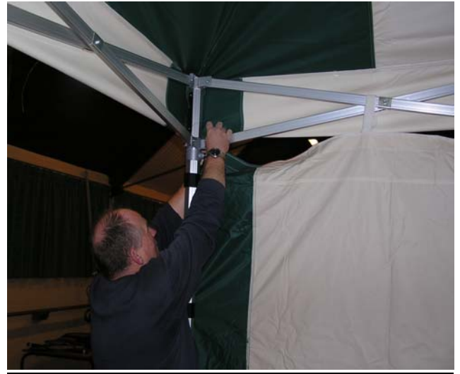
With the legs extended, the windproof side panels are attached.
