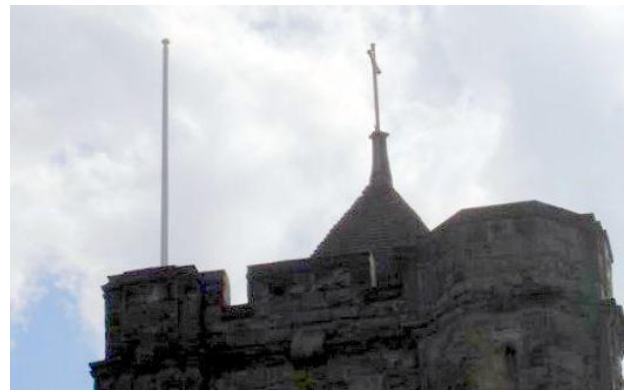
The church tower, complete with flagpole housing antennas for GB3MH and GB7MH
